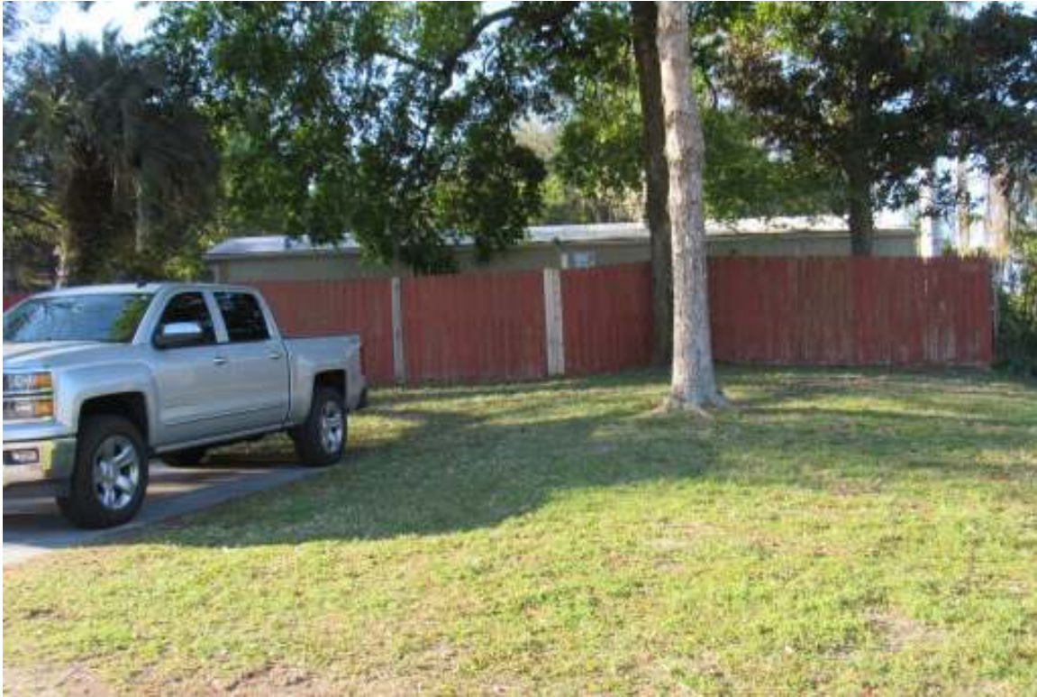
View of required perimeter fence along north property line
